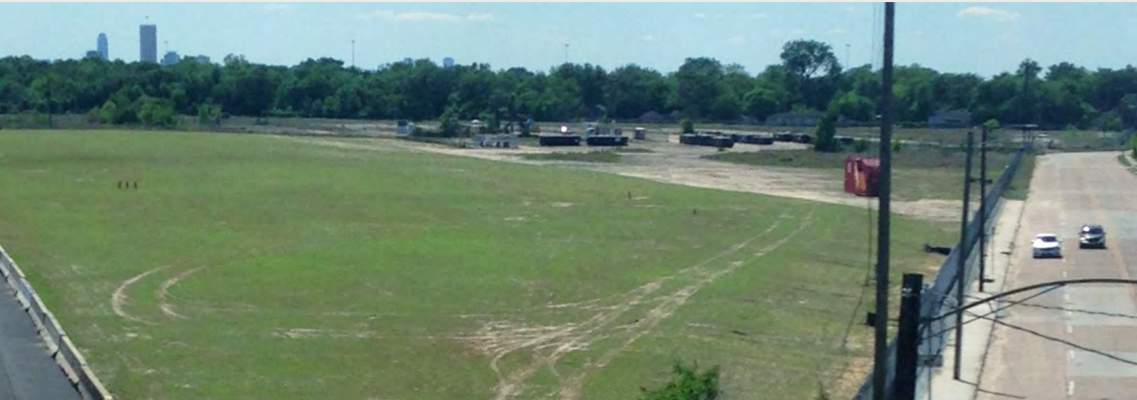
Soil cap at former HWPW Site. Sidewalk concrete cap along Liberty Road constructed in 2016.
