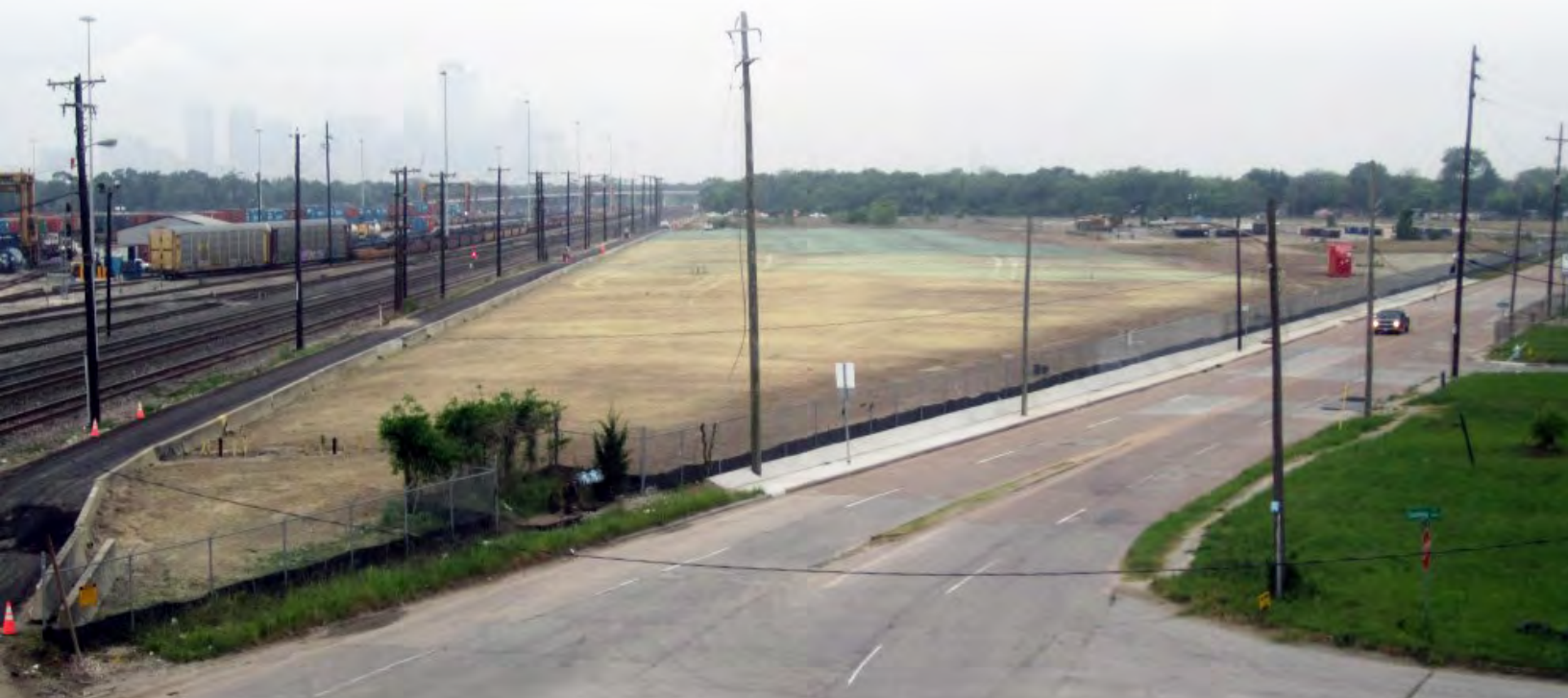
Soil cap at former HWPW Site. Sidewalk concrete cap along Liberty Road and asphalt cap constructed in 2016.
