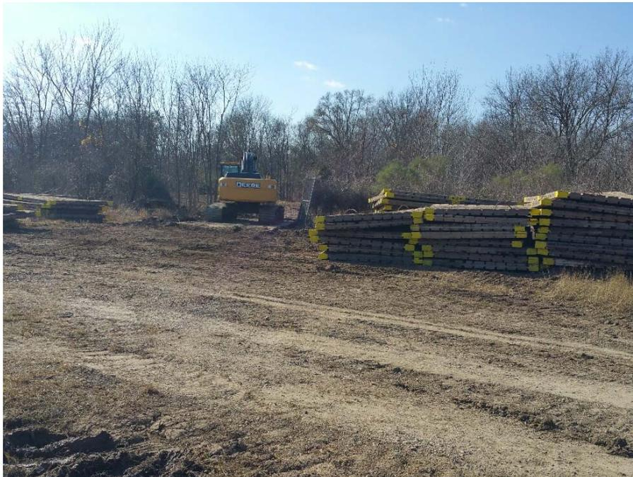
**Photograph 12: Wooden mats being laid out for access to Areas D, E and F (1-23-2016).**
