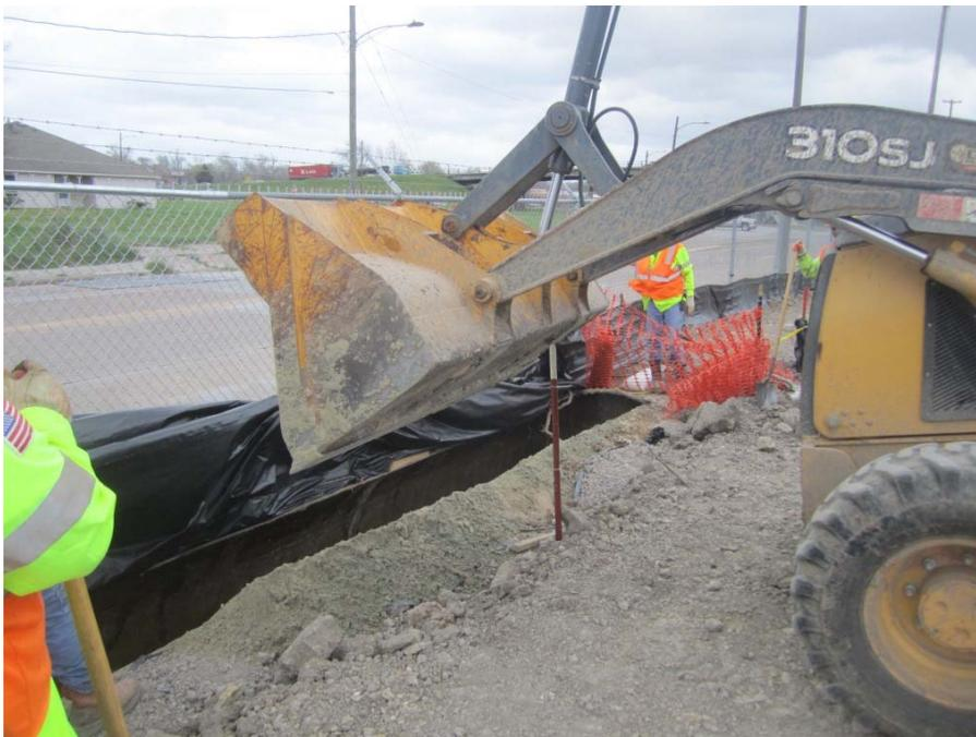
**Photograph 58: Placement of cement-stabilized sand within the cleaned out oil/water separator (3-11-2016).**
