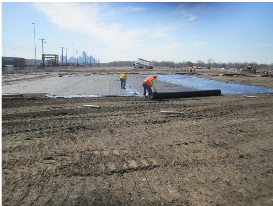
**Photograph 51: Placement of vapor barrier and geotextile fabric on Soil Cap Area, viewing W (2-29-2016).**
