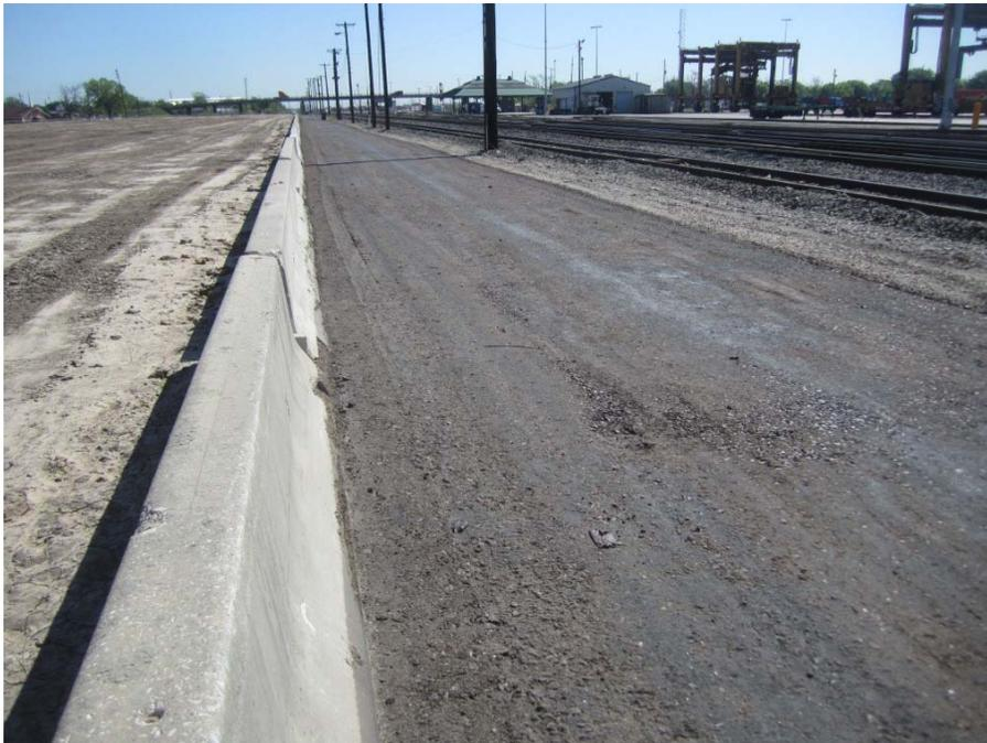
**Photograph 70: Asphalt Cap access roadway with prime coat applied and ready for paving (4-8-2016).**
