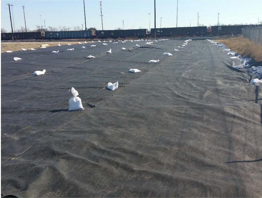
**Photograph 31: Installation of vapor barrier and geotextile fabric on consolidated soils within Cap area (2-4-2016).**
