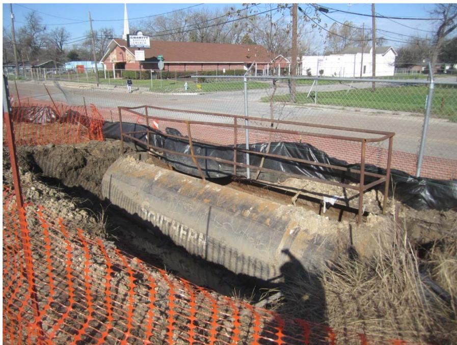
**Photograph 9: Excavation of soil from around oil/water (railcar) separator (SWMU 11)
