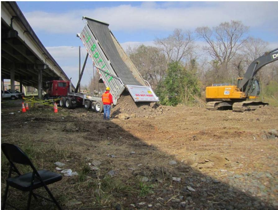
**Photograph 40: Unloading of clean backfill material for Area G (2-17-2016).**
