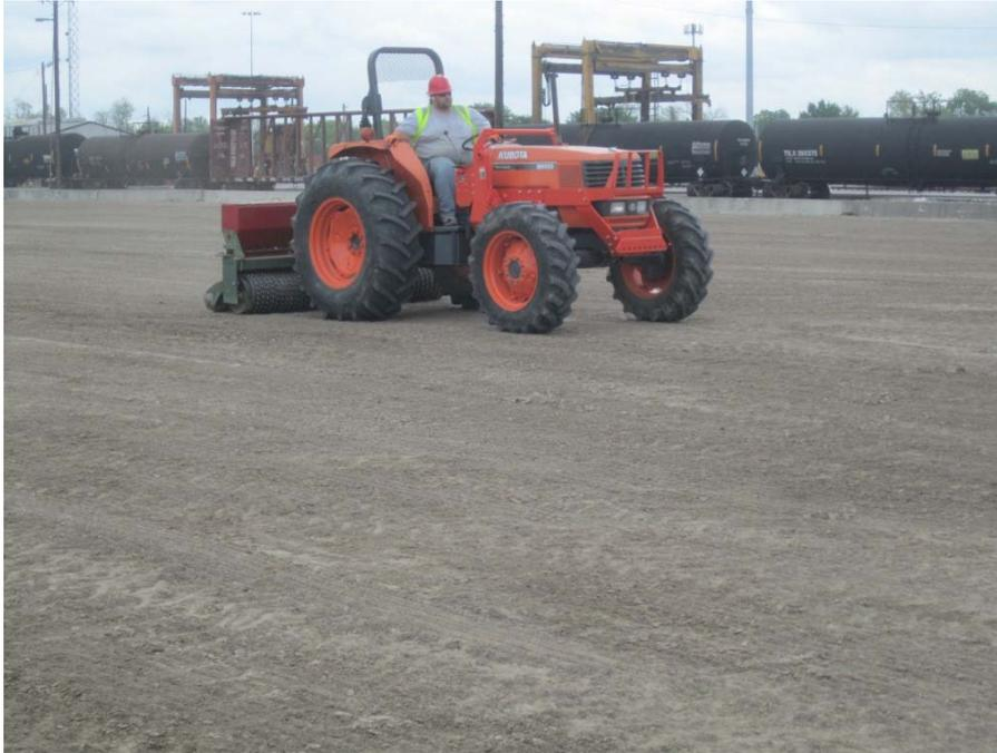
**Photograph 71: No-till drill seeding of Soil Cap Area (4-8-2016).**
