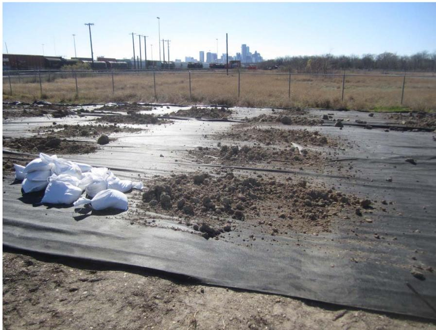
**Photograph 33: Use of clean soil for holding vapor barrier and geotextile fabric in place (2-11-2016).**
