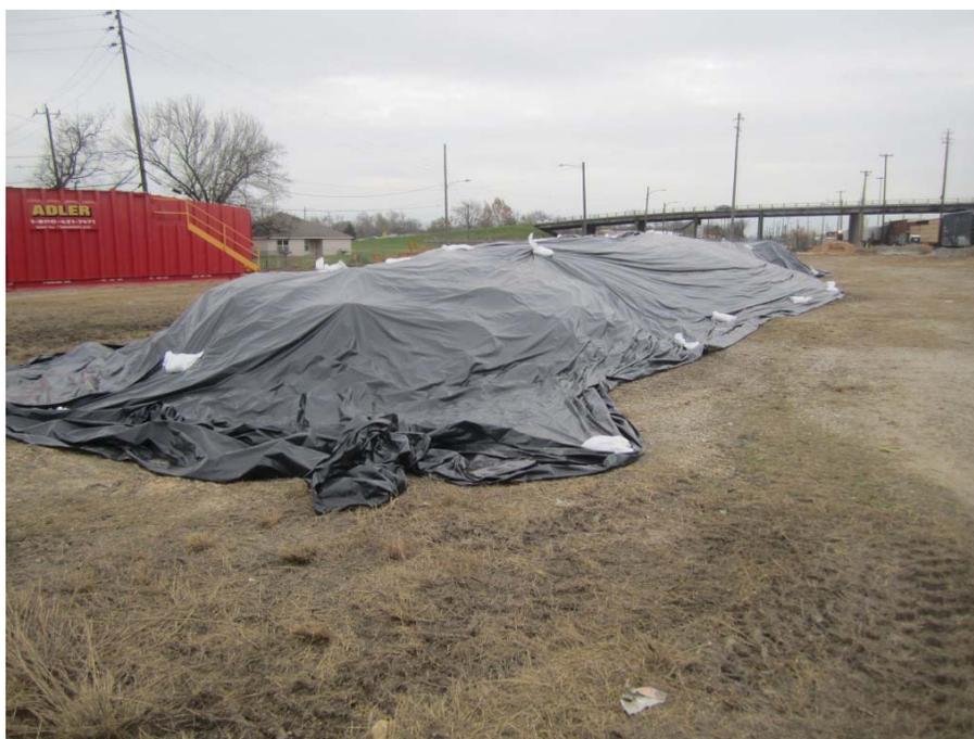
**Photograph 10: Covered stockpile of excavated soil from sidewalk area and near oil/water
