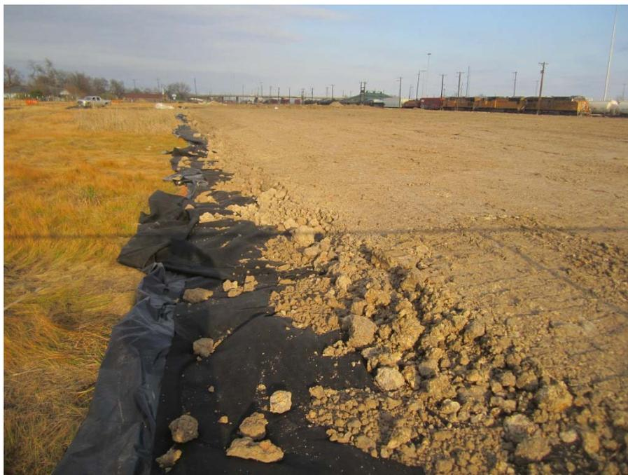
**Photograph 41: NW corner of Soil Cap Area with vapor barrier, geotextile fabric and 12-inches of clay cover, viewing NE (2-18-2016).**
