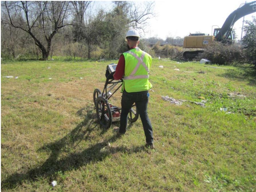
**Photograph 36: Utility locate using ground penetrating radar prior to excavation of Area G (2-13-2016).**
