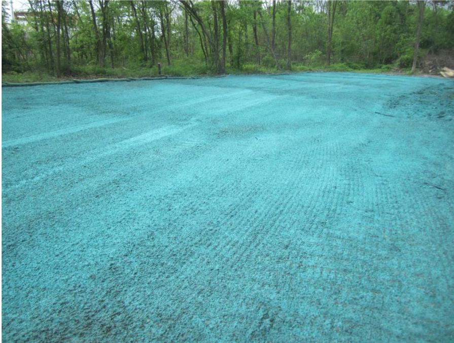
**Photograph 73: Completion of hydromulch of Area F (4-8-2016).**
