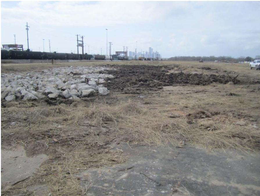
**Photograph 14: Concrete rubble from (SWMU 8) and shredded vegetation placed within bottom of cap (1-29-2016).**
