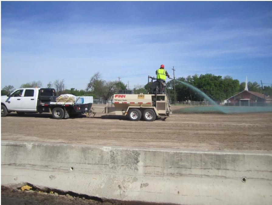
**Photograph 74: Hydromulch application on Soil Cap Area (4-11-2016).**
