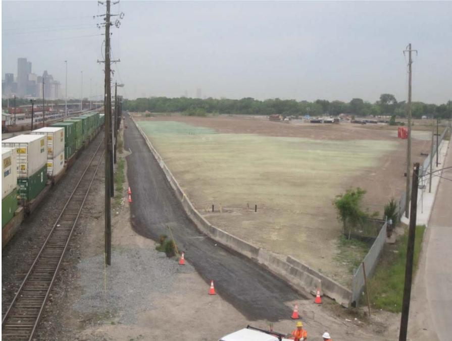
**Photograph 77: Hydromulch coverage on Soil Cap (4-13-2016).**
