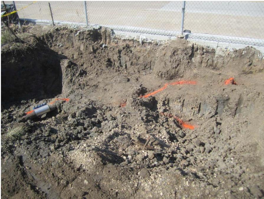
**Photograph 46: Exposed water lines encountered in Area A excavation, just east of railcar (2-25-2016).**
