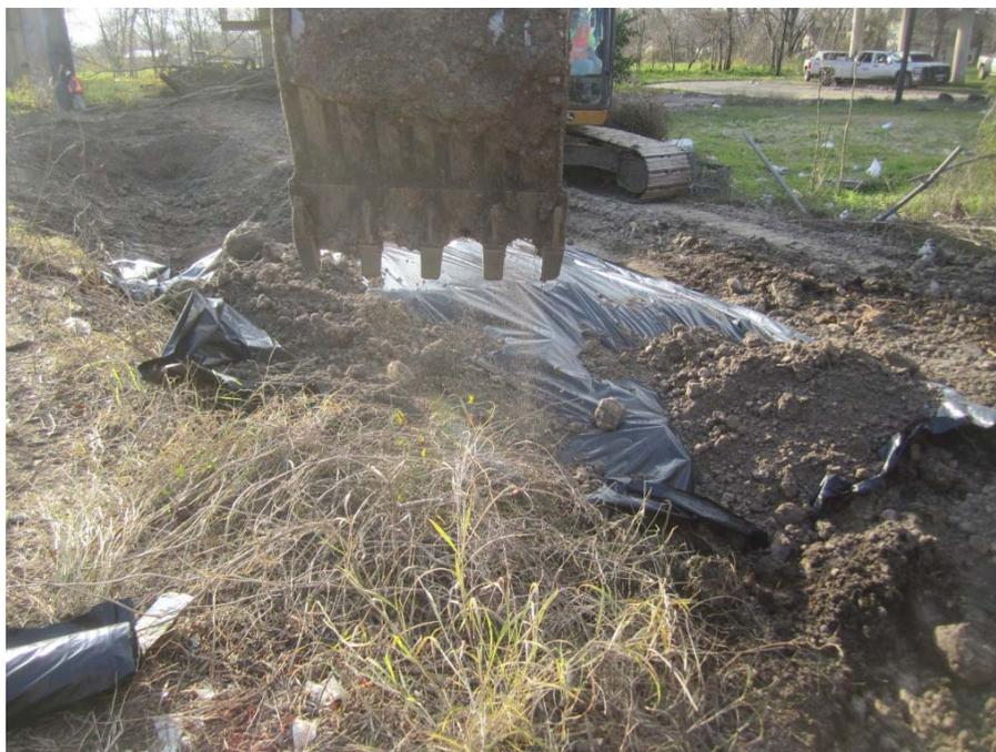
**Photograph 38: Cover stockpiled soils with plastic and clean backfill during overnight hours (2-15-2016).**
