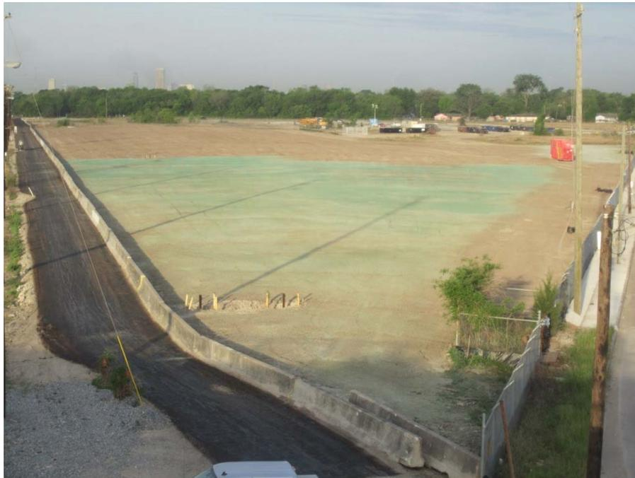
**Photograph 76: Progress of hydromulch on Soil Cap (4-12-2016).**
