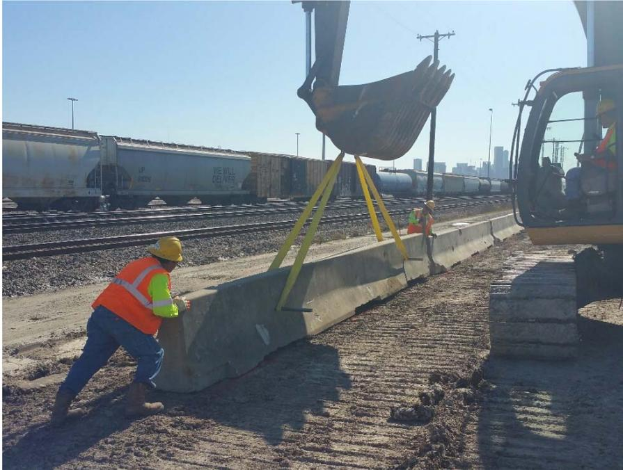
**Photograph 61: Resetting concrete barriers along southern boundary of Soil Cap Area (3-18-2016).**
