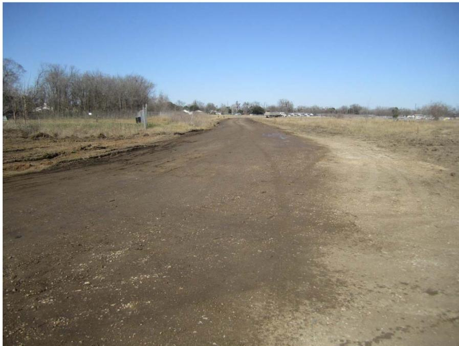
**Photograph 25: Watered haul route to control dust, viewing N (2-3-2016).**
