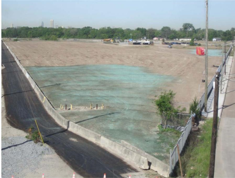
**Photograph 75: Progression of hydromulch coverage on Soil Cap, viewing W (4-11-2016).**
