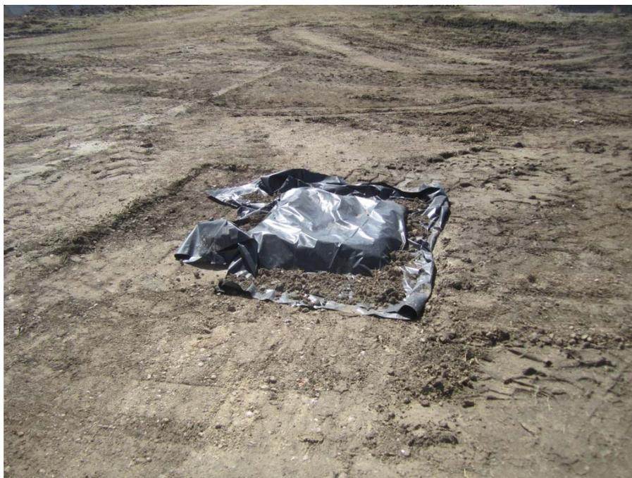
**Photograph 50: Sealing off a storm drain inlet within Soil Cap Area with concrete plug and covered with plastic sheeting (2-24-2016).**
