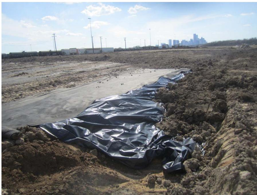
**Photograph 52: Anchor trench for northern boundary of soil cap (2-29-2016).**
