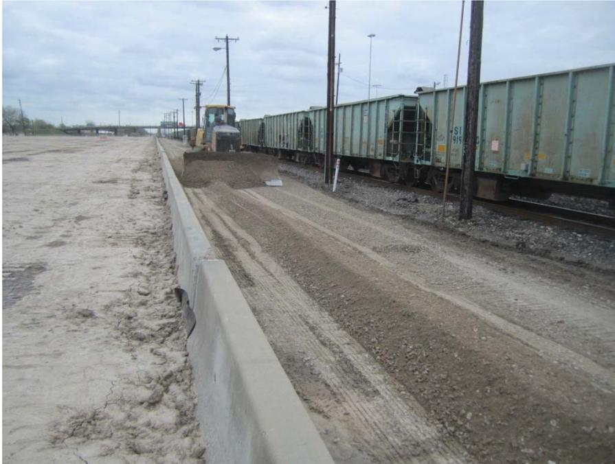
**Photograph 65: Grading of Asphalt Cap Area prior to asphalt paving (3-25-2016).**
