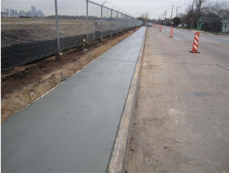
**Photograph 7: Concrete sidewalk cap area, concrete sidewalk poured and finished (1-20-2016).**
