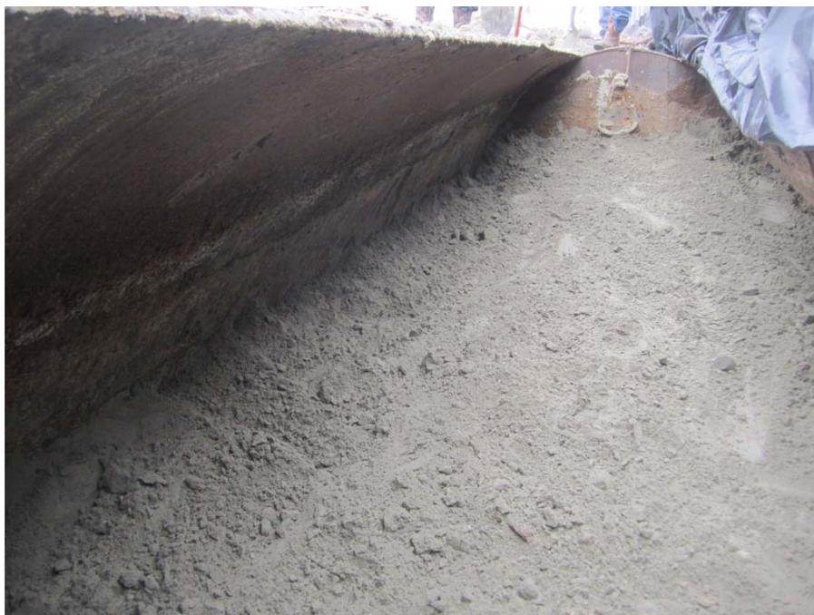
**Photograph 60: Cleaned out oil/water separator being backfilled with cement-stabilized sand (3-11-2016).**
