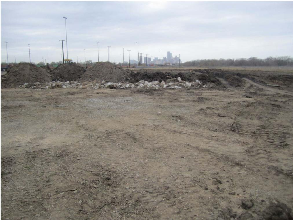
**Photograph 30: Consolidated soil materials being placed within Soil Cap Area (2-3-2016).**
