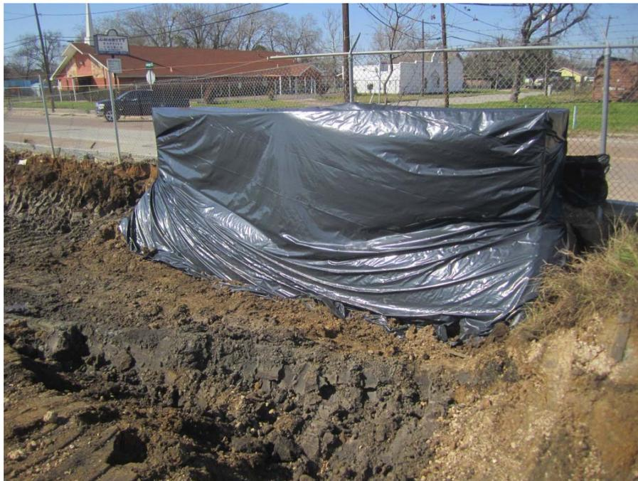
**Photograph 49: Oil/Water separator wrapped in plastic to keep out rainwater and soils during excavation (2-24-2016).**
