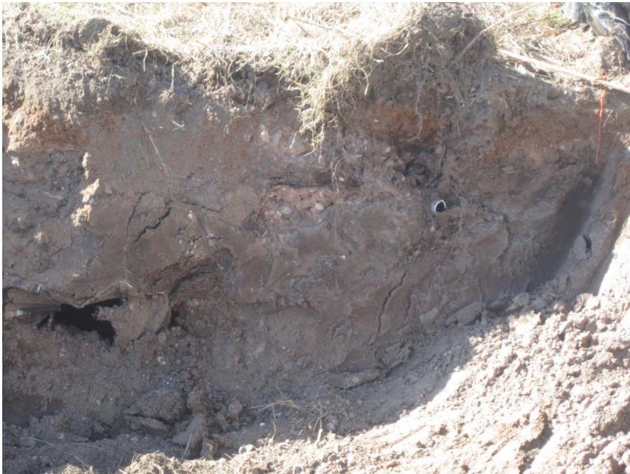
**Photograph 28: Two pipes encountered within Area A excavation. Large pipe (24" CMP) is part of the storm drain system while other pipe (3" PVC) is an abandoned water line (2-4-2016).**
