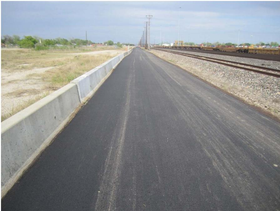
**Photograph 78: Asphalt paving of access roadway Asphalt Cap, viewing NE (4-9-2016).**
