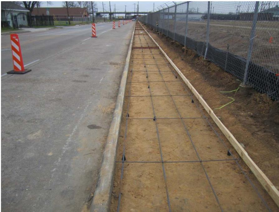
**Photograph 6: Concrete sidewalk cap area, sand bedding and reinforcing steel for concrete sidewalk (1-19-2016).**
