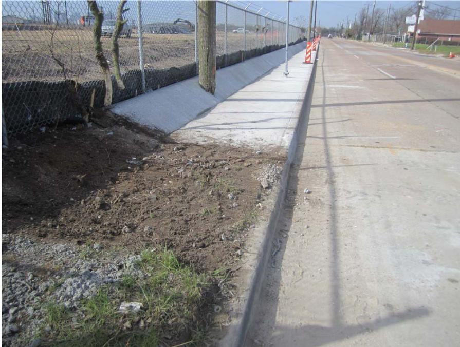
**Photograph 13: Finished concrete sidewalk and side slope area, viewing west (1-29-2016).**
