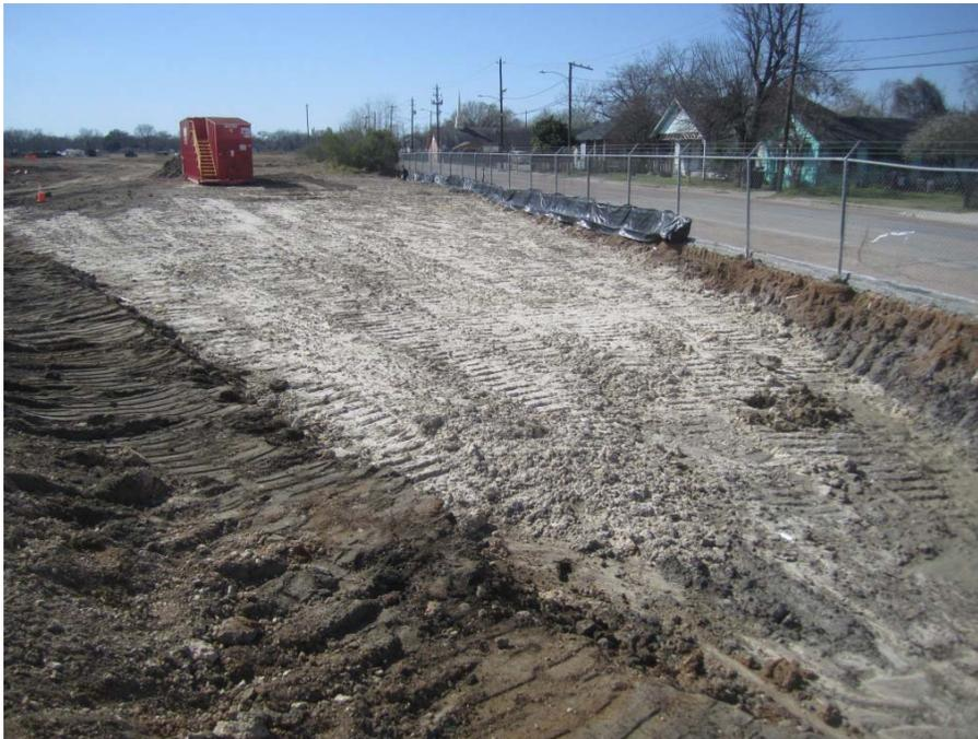
**Photograph 48: Clean backfill material being placed within Area A, viewing W (2-24-2016).**
