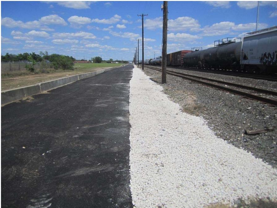
**Photograph 80: Placement of ballast between roadway and rail (4-22-2016).**
