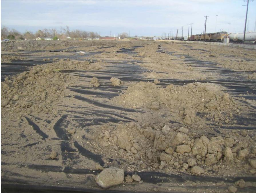
**Photograph 43: Use of clean soil material to hold down vapor barrier and geotextile fabric on soil cap, viewing E (2-19-2016).**
