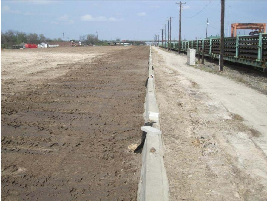
**Photograph 63: Concrete barrier wall making up the boundary between Soil Cap Area and Asphalt Cap (3-18-2016).**
