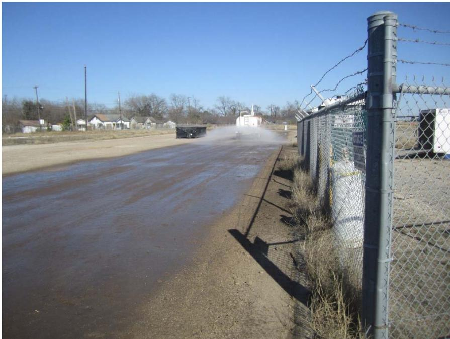
**Photograph 24: Water spray to control dust along haul route (2-3-2016).**
