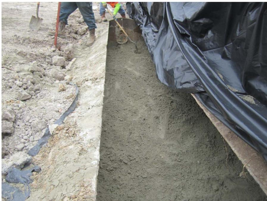
**Photograph 59: Cement-stabilized sand within oil/water separator (3-11-2016).**
