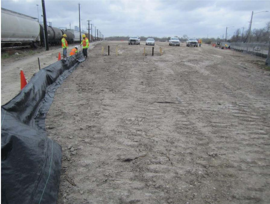
**Photograph 57: Installation of silt fencing on southern boundary of soil cap (3-11-2016).**
