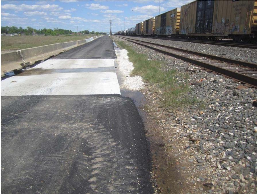
**Photograph 79: Completed concrete low-water crossing (4-22-2016).**
