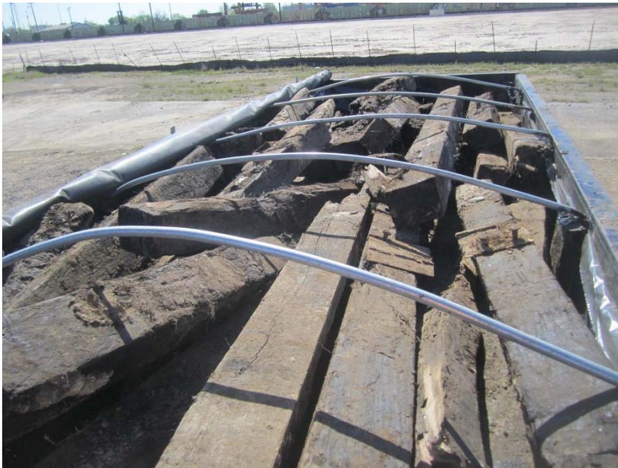
**Photograph 64: Roll-off with weathered cross ties removed from project and ready for disposal at landfill (3-25-2016).**
