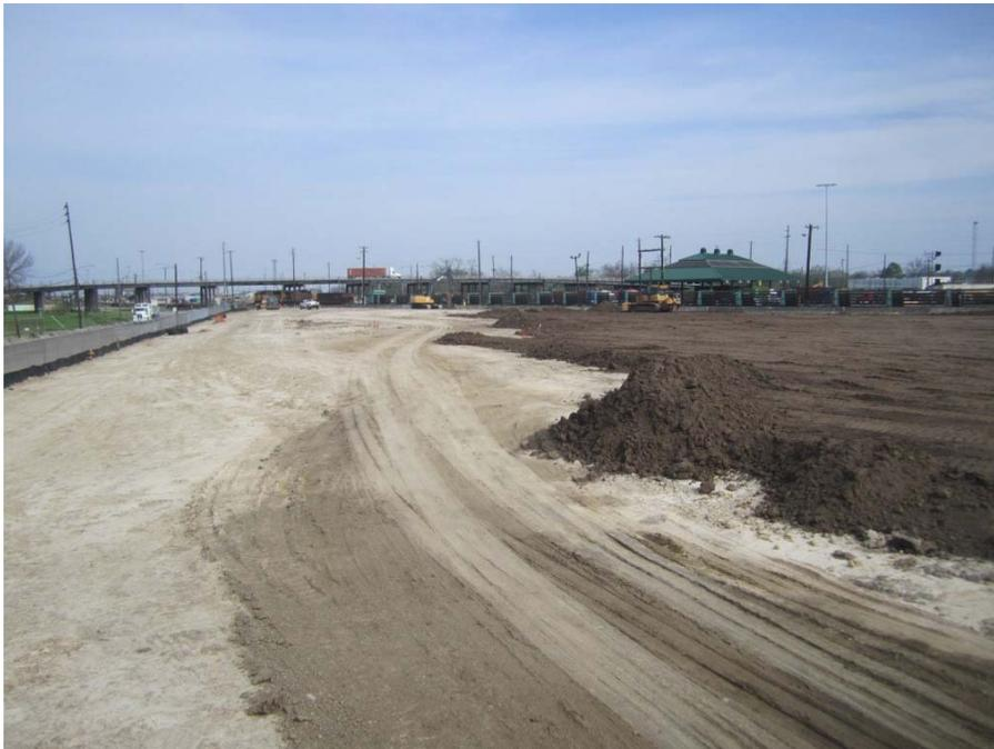
**Photograph 62: Placement of topsoil on Soil Cap Area, viewing SE (3-18-2016).**
